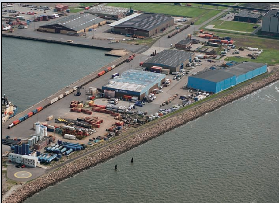
Above is a bird's-eye view of the Jutlandia transloading base in Denmark. CSPI has been shipping flow improver products through Jutlandia for more than 20 years.
